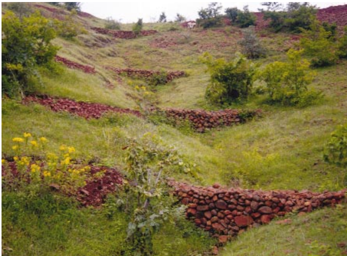
Gully Plugs, Nagzari Village, (Oct. 1999). Photo: WOTR
