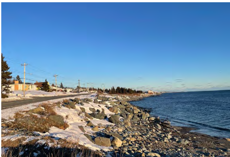
Figure 5. Shore Road, before the Building With Nature Project
