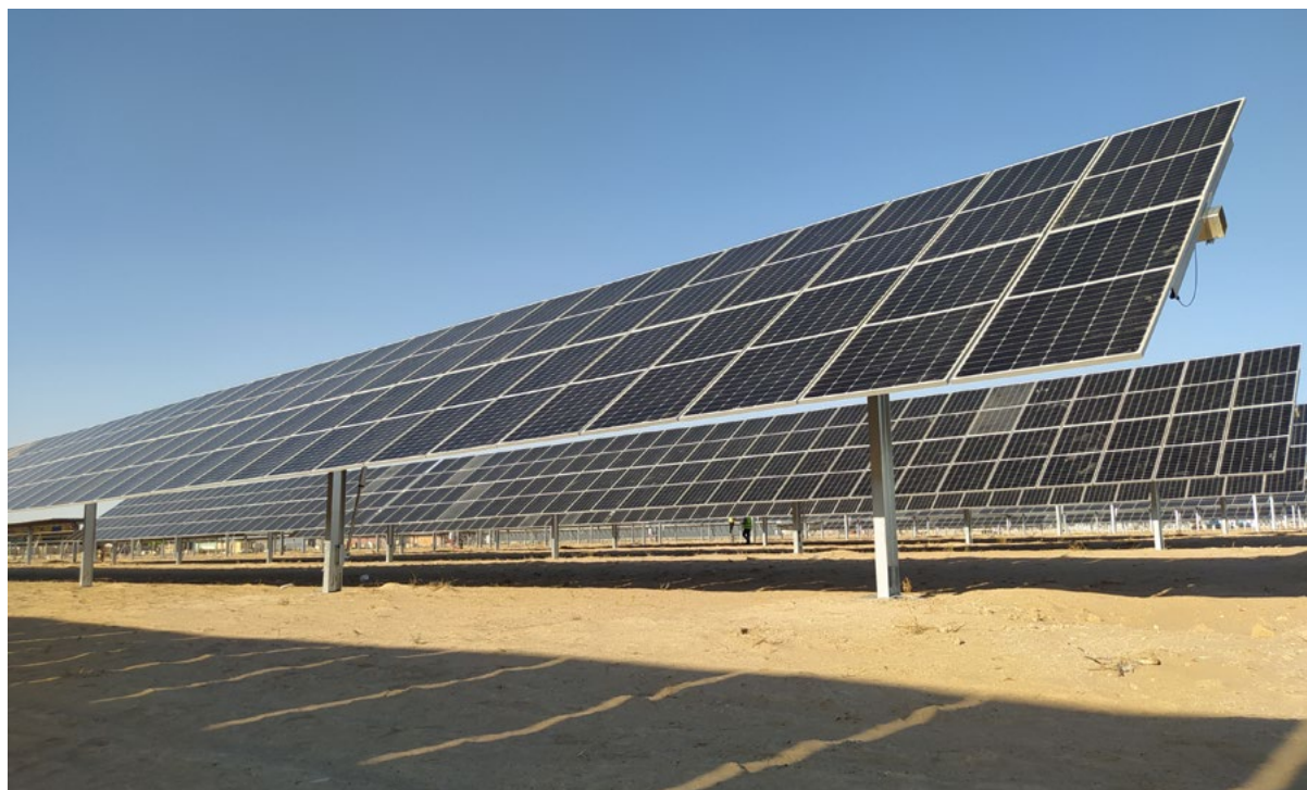
Figure 14. Solar panel installation
